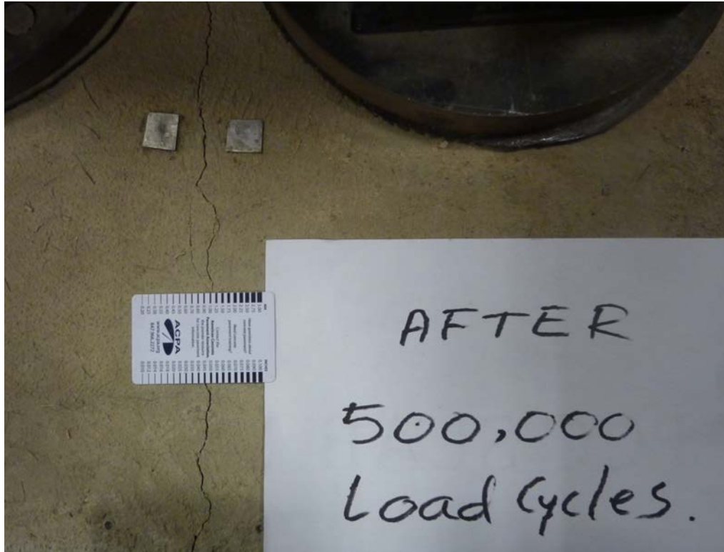
Figure 5.61. Crack after fatiguing for FRC1 slab, top view.
