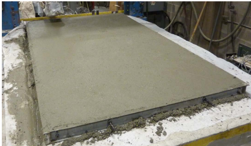
Figure 3.29. Example of a finished slab.
