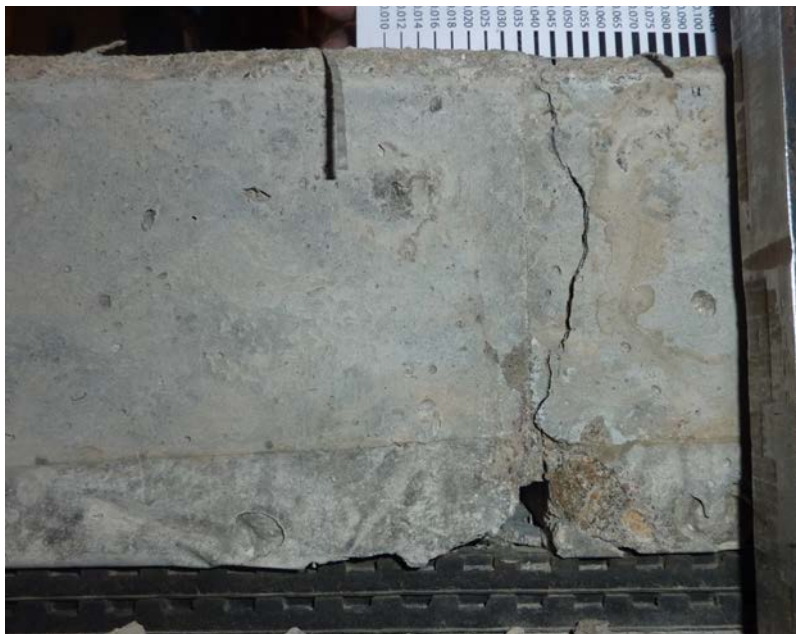
Figure 5.68. Crack profile near the loading location for the FRC2 slab, side view.
