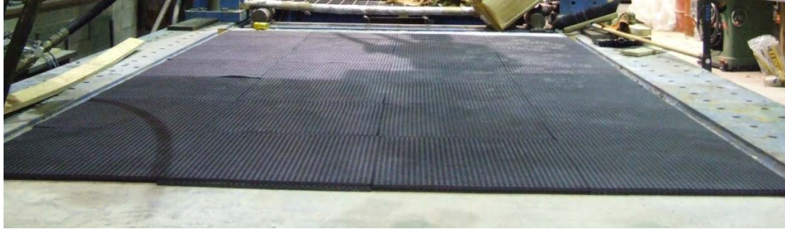
Figure 3.24. Two layers of Fabel 25 laid on the concrete foundation.
