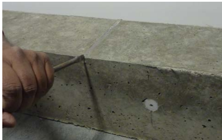
Figure 3.18. Removal of cracking bar from the concrete.
