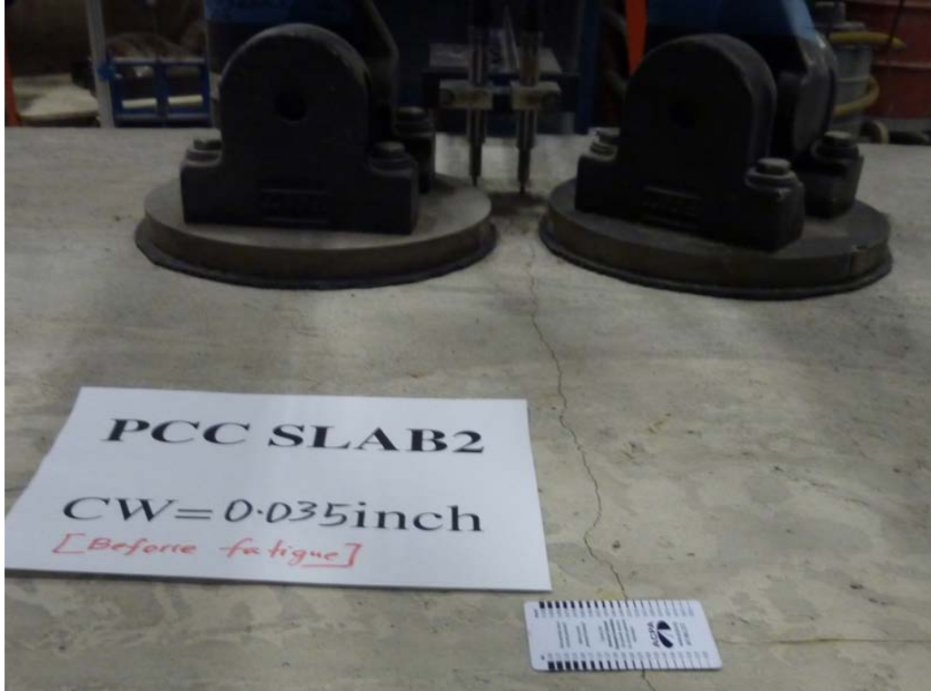
Figure 5.52. Picture of the crack before fatiguing.
