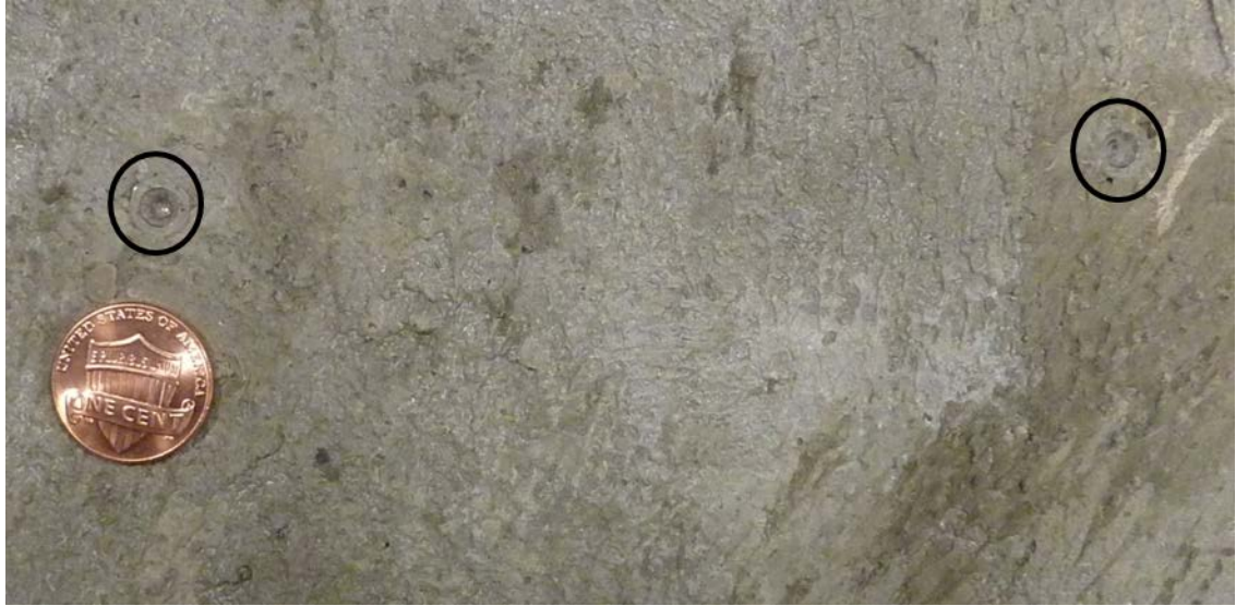
Figure 3.30. Photograph of a pair gage studs inserted into the concrete.
