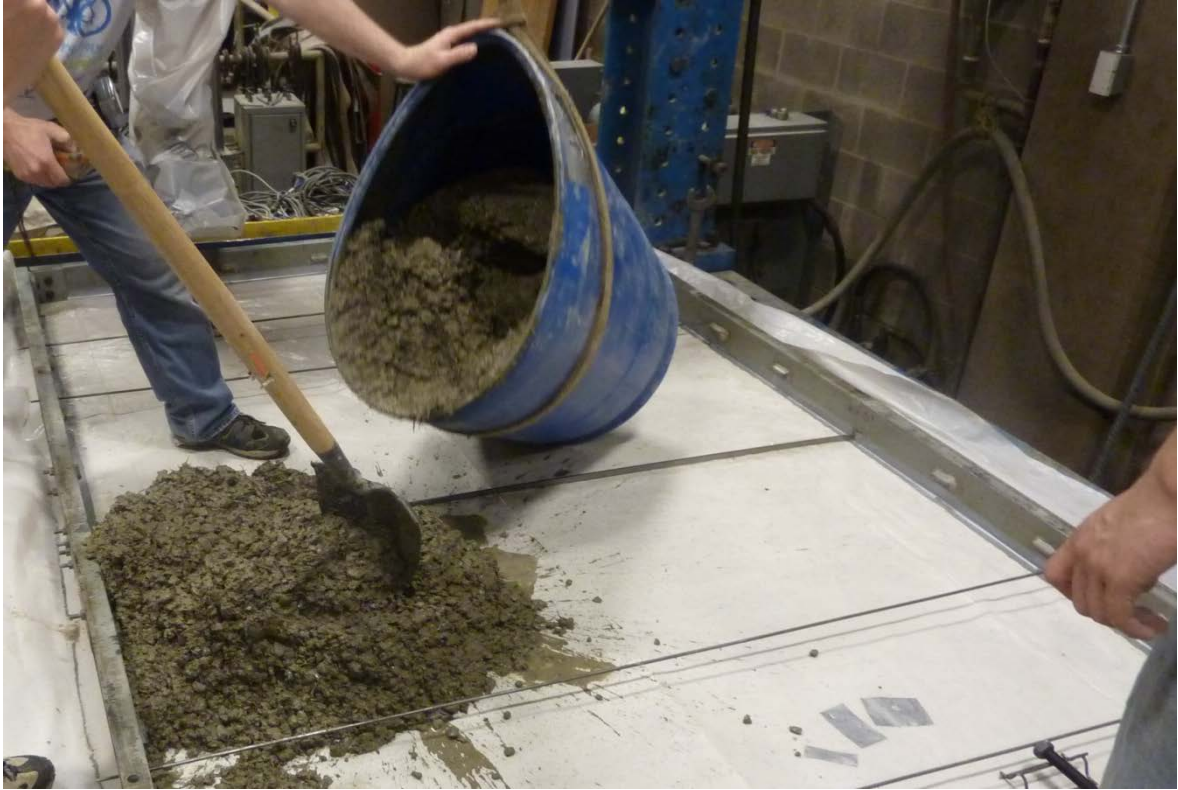
Figure 3.28. Casting of the slab.
